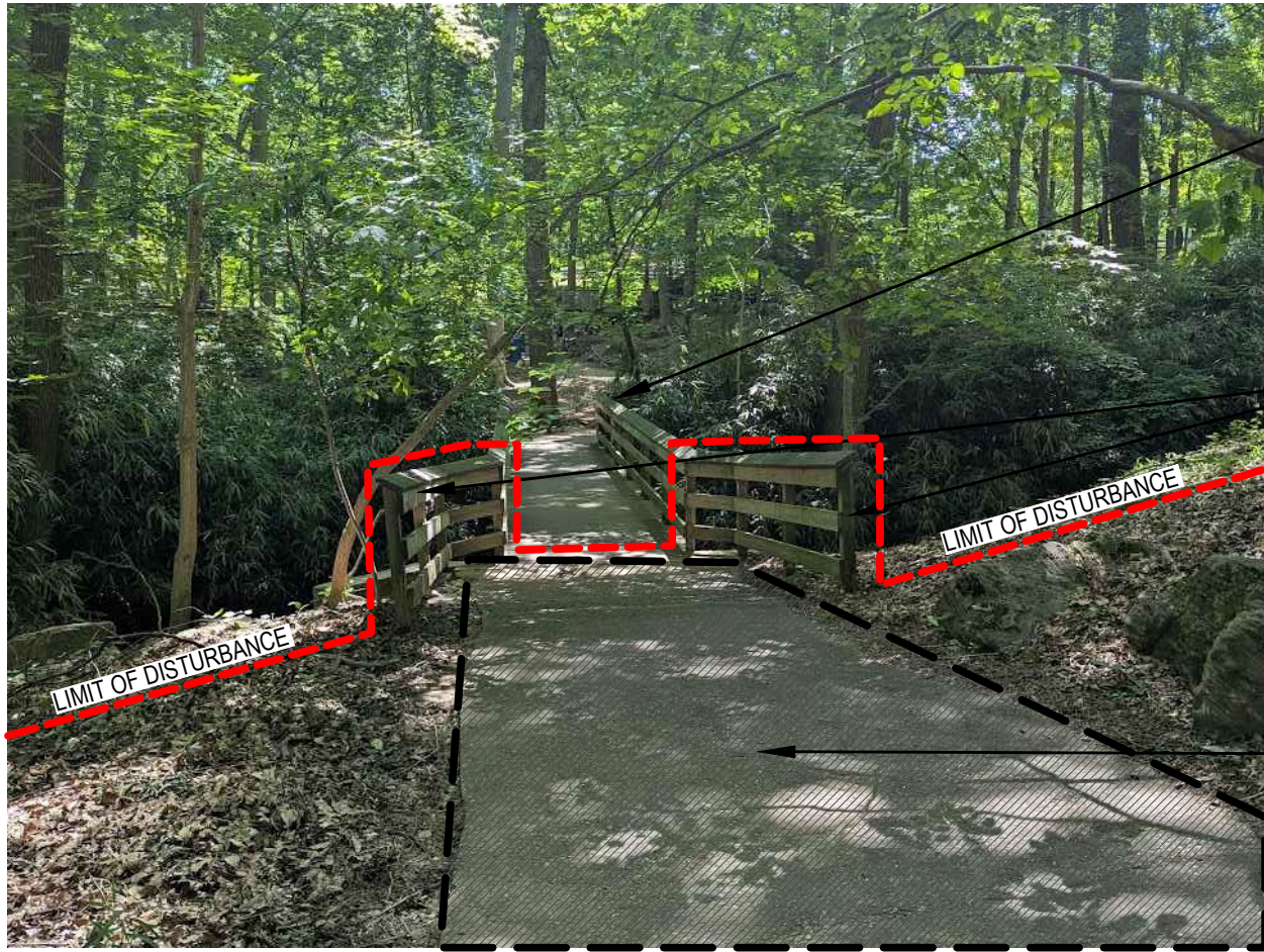
4 EXISTING BRIDGE B - IMAGE NOT TO SCALE
