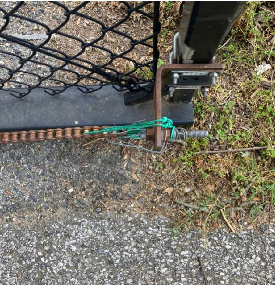
Broken chain-plate on Gate 18.
