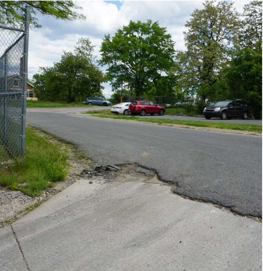
Damaged paving that needs patching.
