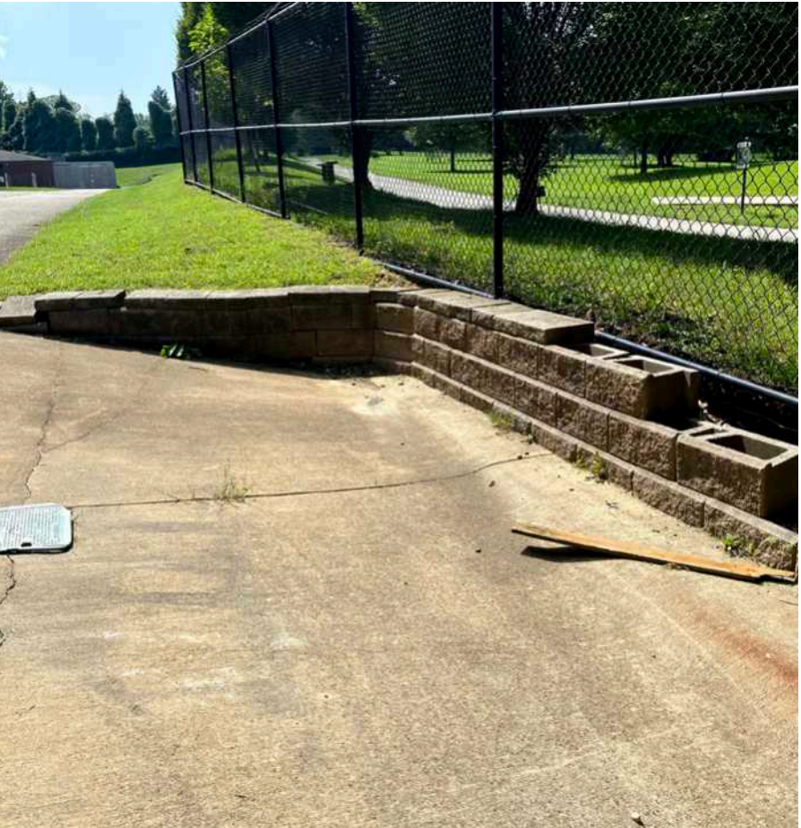
Existing retaining wall with missing cap blocks.
