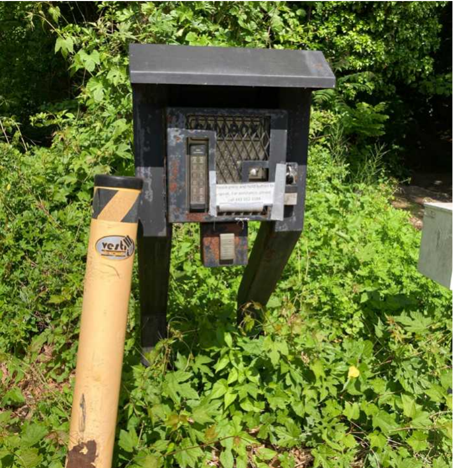
Detail view of outdated call box - rusty and in poor condition.
