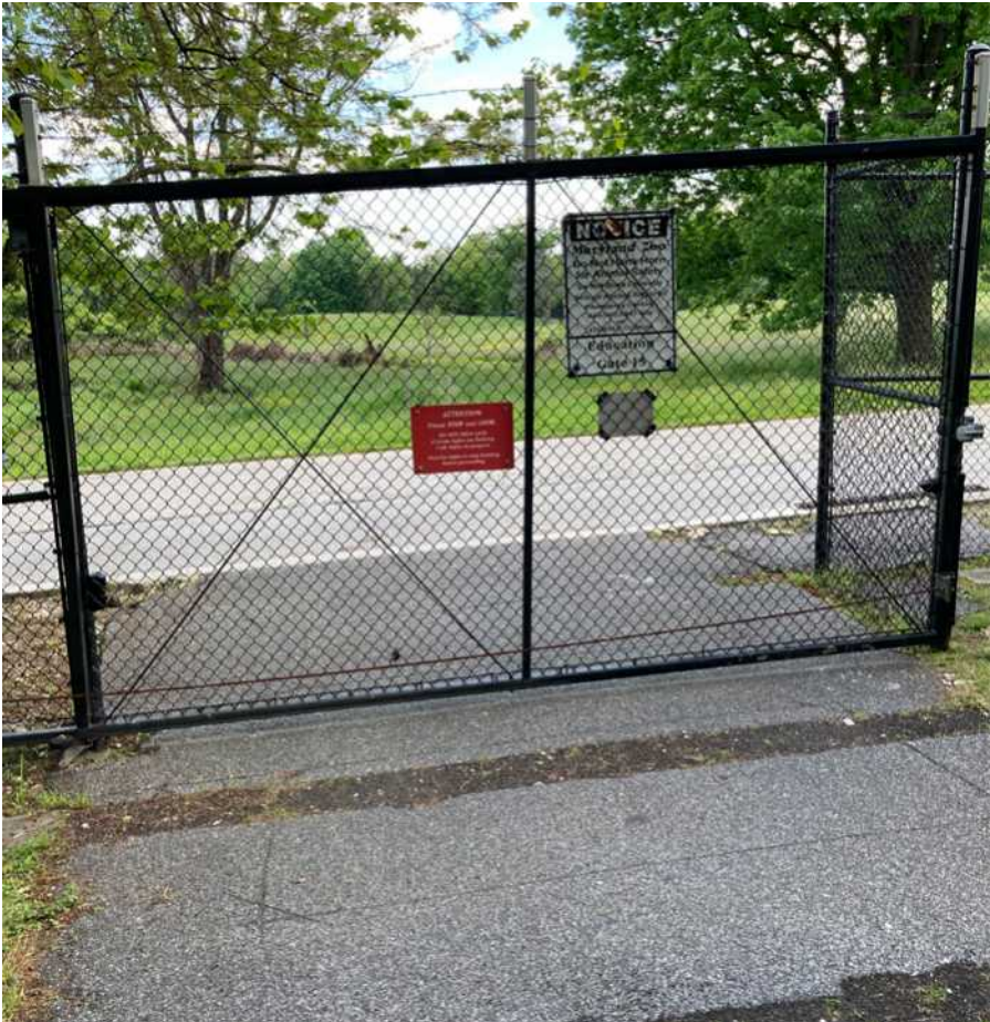
Elevation view of Gate 15. Set at an angle matching paving.
