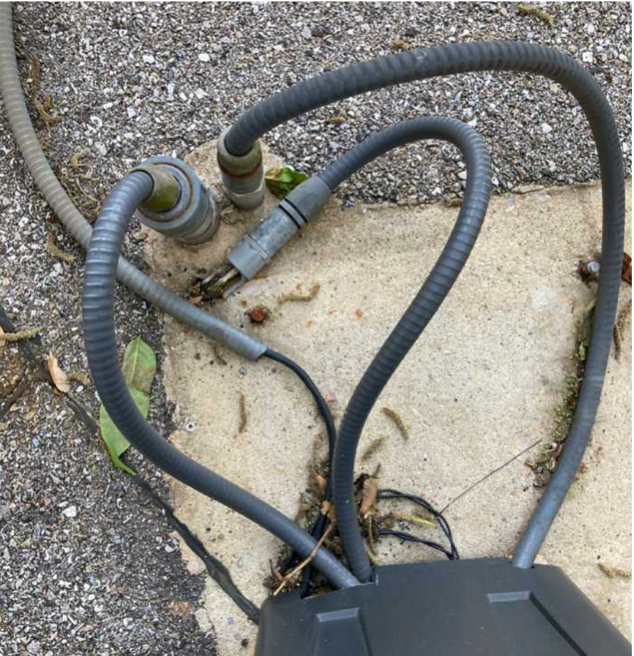
Gate 11 electrical cables are damaged.
